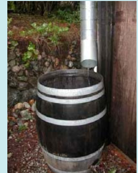
Simple rainwater collection system
